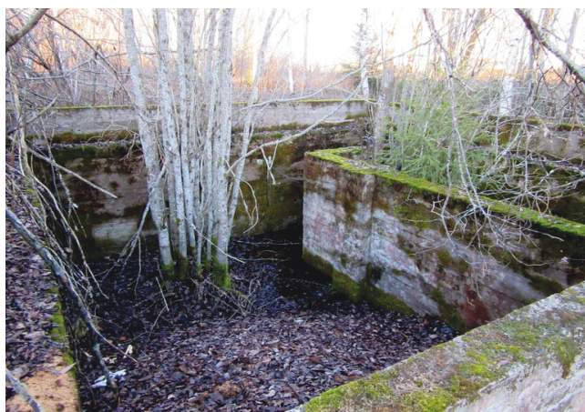
Kohde no. 2, betoniperustus.
